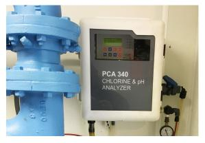
chlorine and pH. Hanna's process chlorine analyzers (PCAs) use the EPA approved DPD method for chlorine measurement and an in-line pH electrode. Currently, KK&W has seven Hanna PCAs in service throughout their municipality, which have proven to be accurate and reliable over the years. These PCAs are linked to a SCADA system
